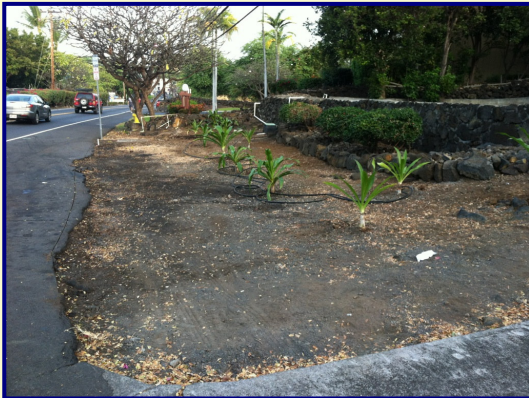
Work Underway at Alii Drive and Walua Road
