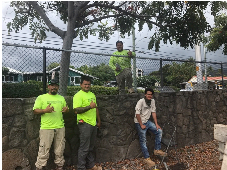
Repairing and replacing the fence fronting the public County Parking Lot
