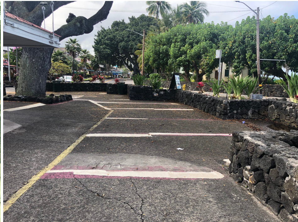
Mahalo to the County of Hawaii Department of Public Works for completing sidewalk repairs at Emma's Square.
