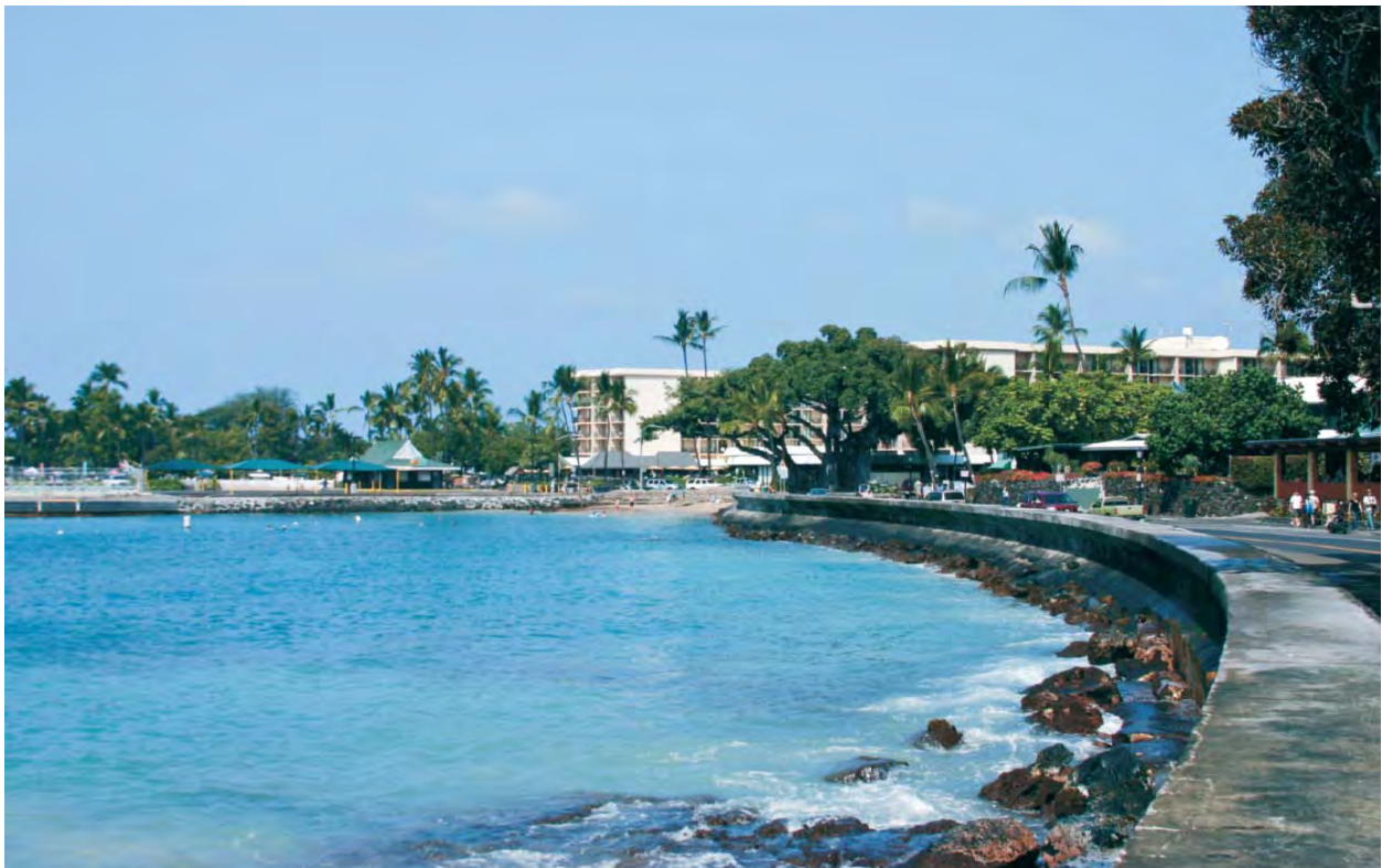
Kailua Seawall (Local Byway Committee photo)
